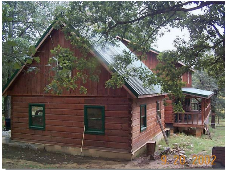
Rear Elevation from Double Garage End
